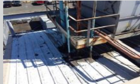
Mechanical room penetrations
